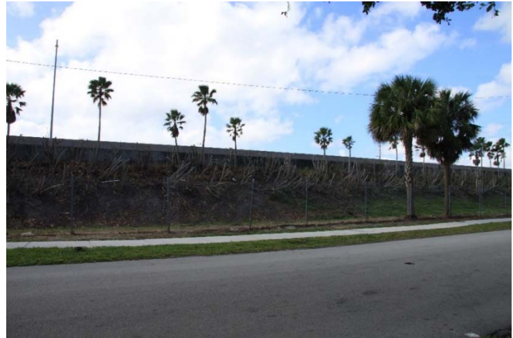
Figure 24 | View from NW 21 st Ave Looking West at I-95
