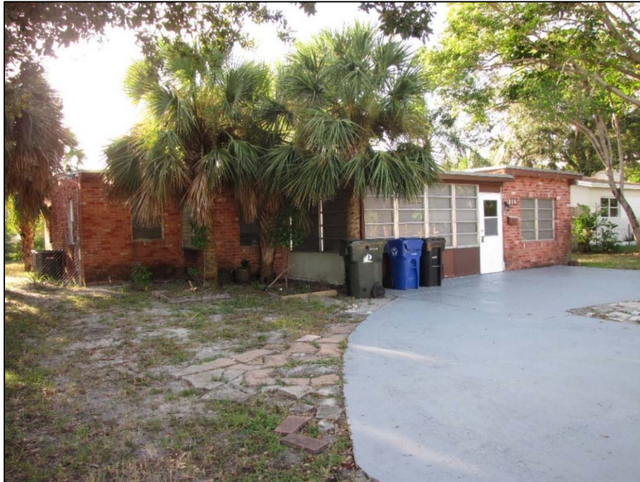
Figure 39 | 109 SW 21 st Way (8BD6777), c. 1953, facing West, exhibits enclosed carport and porch, replaced windows and doors, northeast corner addition
