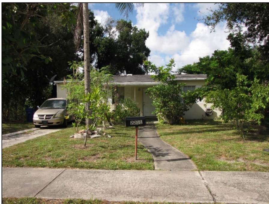
Figure 11 | 2211 SW 1 st Court (8BD6749), c. 1953, facing North, exhibits enclosed carport, replaced windows and doors, and a north side addition
