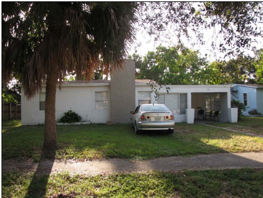
Figure 33 | 139 SW 21 st Way (8BD6771), c. 1953, facing West, exhibits enclosed portion of carport, replaced windows and doors
